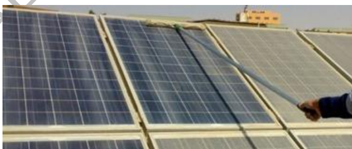
Figure 18 An example of heavy dust deposit
