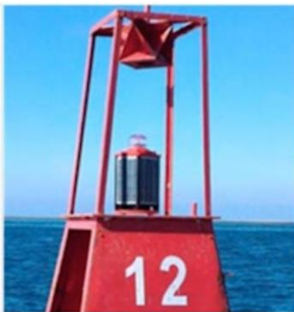
Figure 25 Examples of shadowing on buoys
