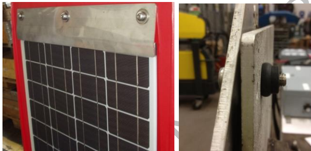
Figure 20 An example of direct fixing.
